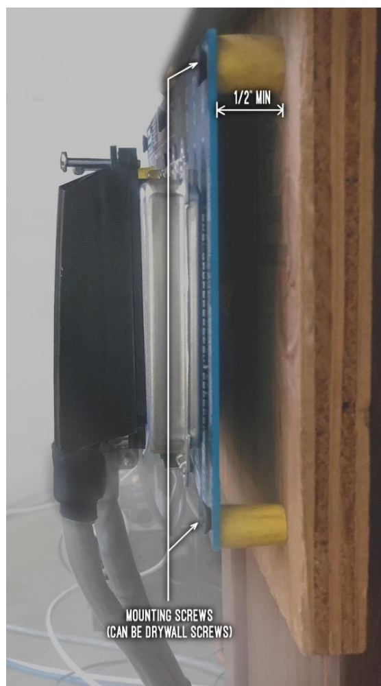
Fig. 6 – KSU Mounted to backboard, office installation.
