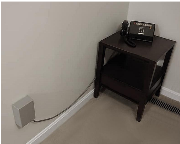
Fig. 49 – 66E3-25 wall installation with decorative cover for a 2830 desk set.
